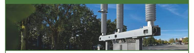
SHE Transmission continues to lead the way in the uptake of alternatives to SF<sub>6</sub> on the transmission network. We have completed an evaluation of the Siemens Blue live tank 132kV circuit breaker concluding it is suitable for use at our Dunbeath substation. We have now successfully completed the Factory Acceptance Test and the circuit breakers will be installed in August 2019.
