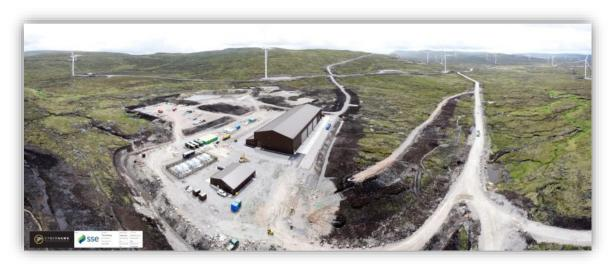
Stronelairg Indoor 132/33kV AIS Substation (energised 24 March 2018) adjacent to the 227.8 MW Stronelairg Windfarm
