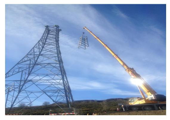
BBK - erecting a new tower on the 275kV line
