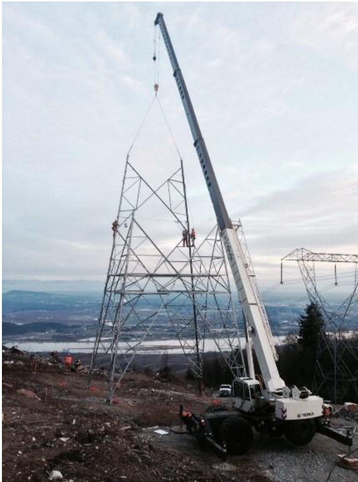
Plate 3.2: Illustrative Image of Steel Lattice Tower Construction
