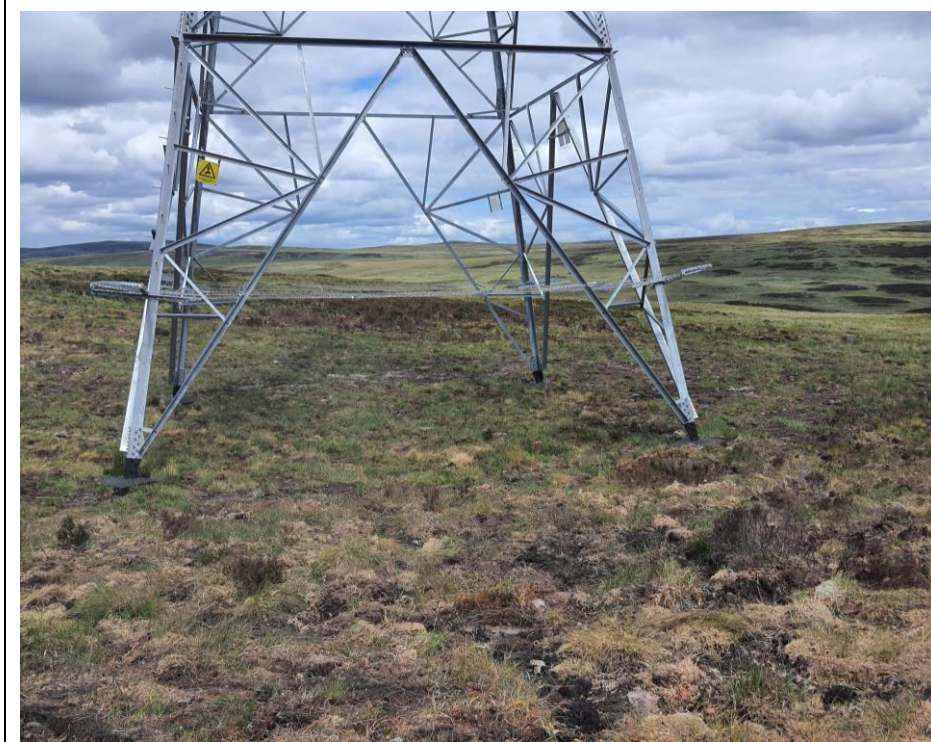
Photo 2: Example of reinstatement around tower foundations.
