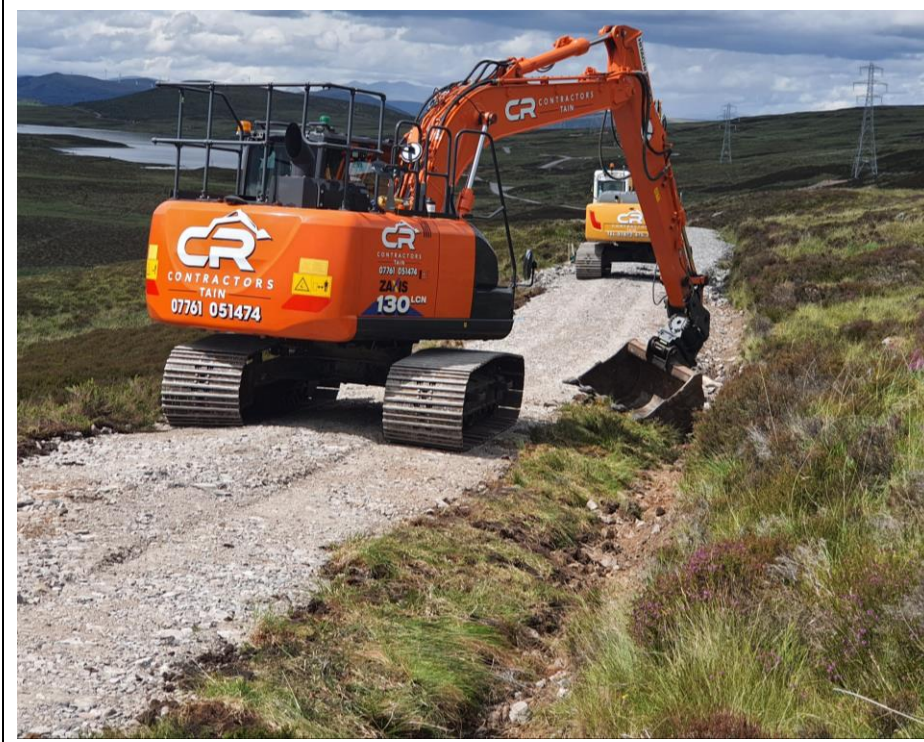
Photo 4: Formation of an access track verge using whole turves.
