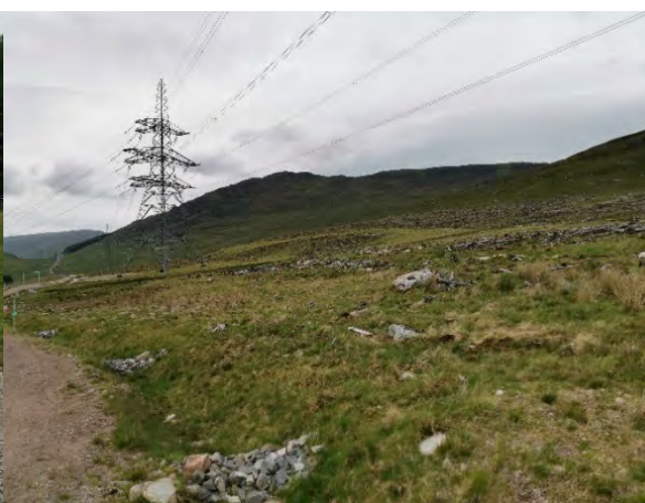
Photo 4: View from Melgarve substation, looking southeast to where Route Option C2B would join Route Option C1. Beaully - Denny OHL visible in picture.
