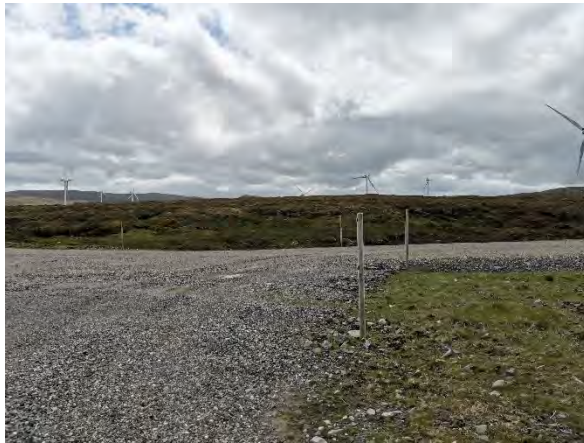
Photo 1: View from Stronelairg Wind Farm facing south in the direction of where Route Option C3 travels east.
