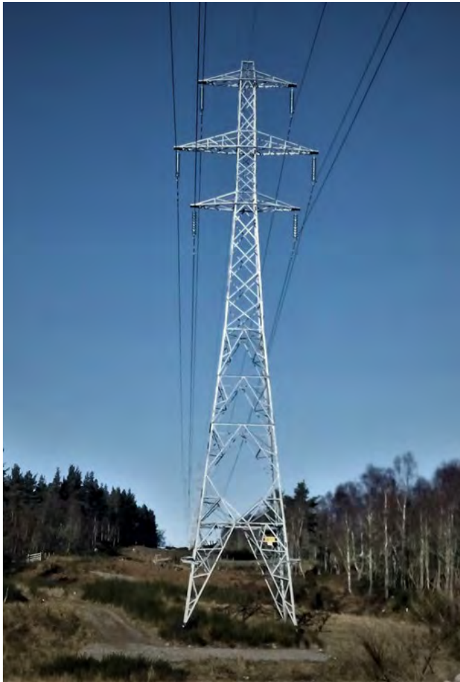
Plate 2.1: Example Steel Lattice Tower OHL Structure
