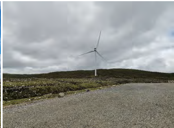
Photo 2: View from Stronelaig Wind Farm on-site substation facing south in the direction of where Route Option D2 travels south towards Glenshero substation.
