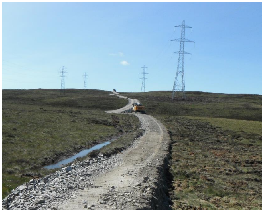
Photo 6: Example of ongoing narrowing works to access track using stored turves.
