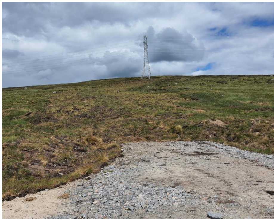
Photo 5: Reinstatement of temporary access track to tower and narrowing and reinstatement around permanent access track.
