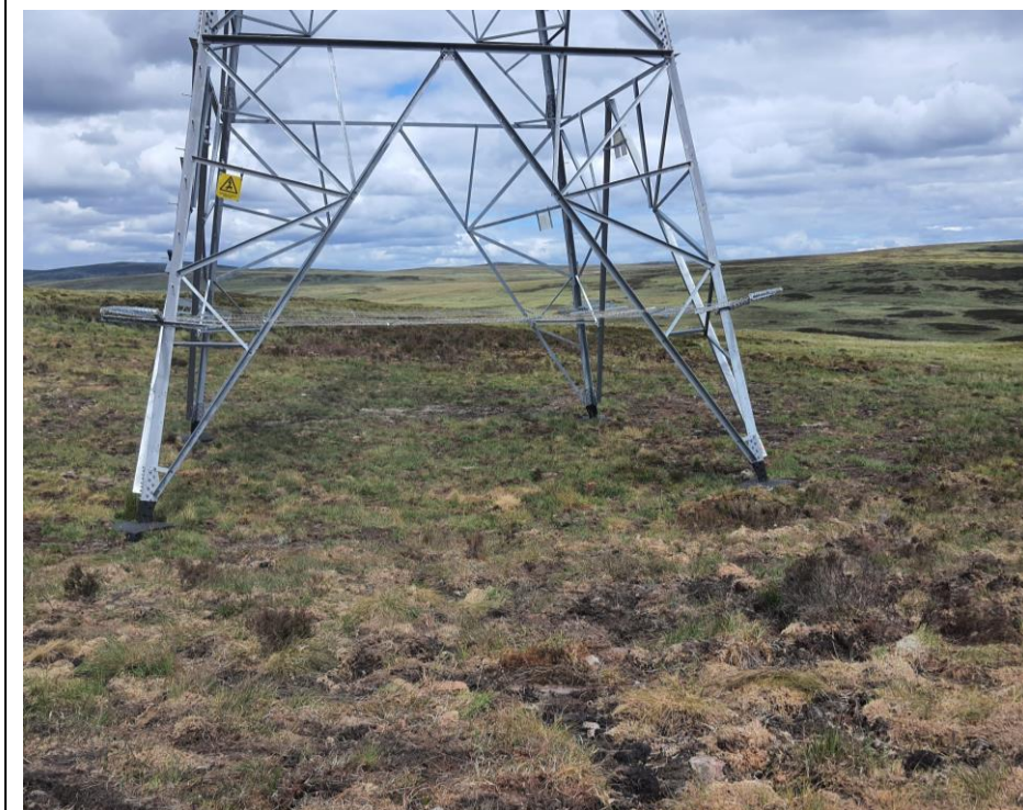
Photo 2: Example of reinstatement around tower foundations.
