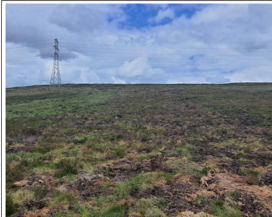
Photo 1: Reinstatement of temporary track using turves.
