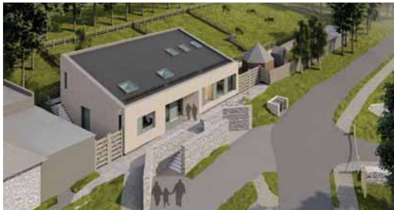
EXCITING NEW ERA: The proposed local larch wood clad building will be around 16 metres by nearly 10 metres but one of the challenges will be building into the site's slope.
