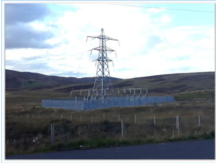
Plate 2.2: Typical Cable Sealing End Compound
