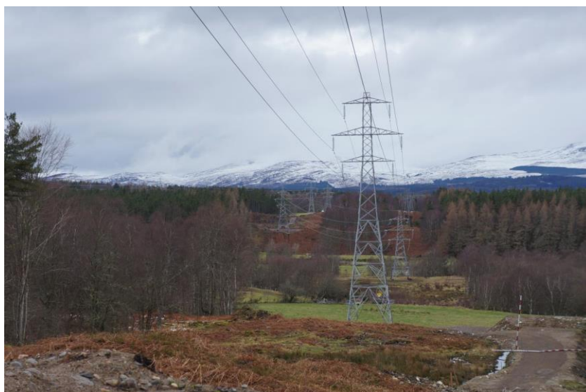
Plate 2.1: Photograph of Steel Lattice Tower Double Circuit (L7 series)
