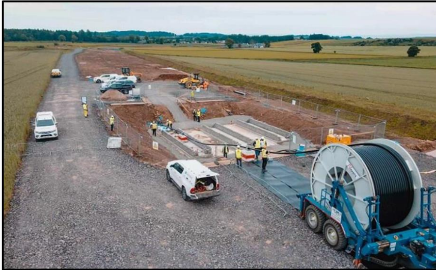
Plate 3.4: Photograph of Underground Cable Installation
