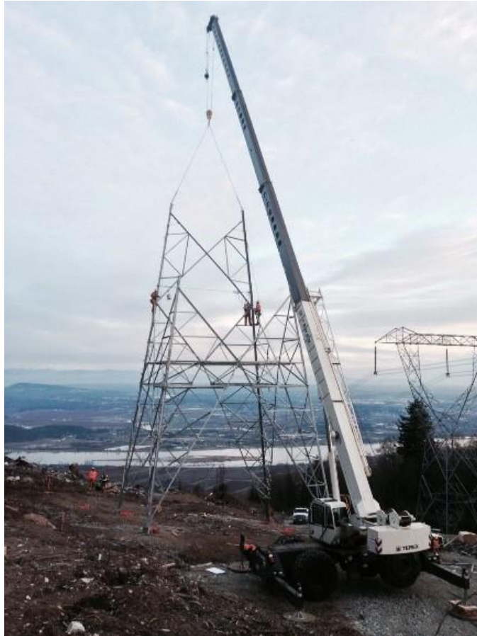
Plate 3.3: Illustrative Image of Steel Lattice Tower Construction
