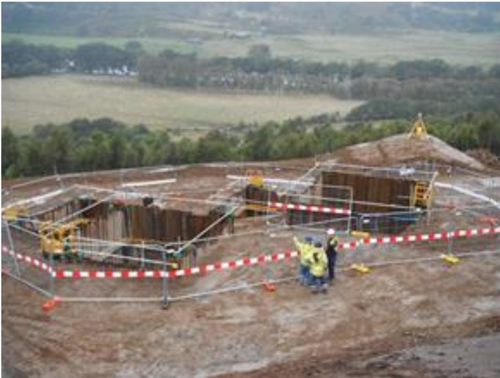
Plate 3.2: Illustrative Image of Tower Foundation Construction
