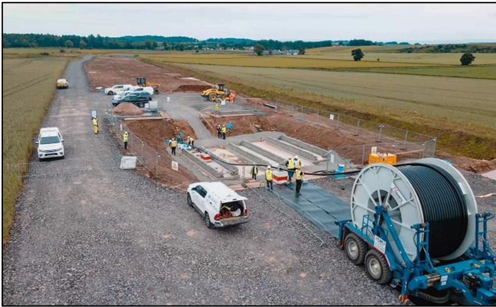
Plate 3.6: Photograph of Underground Cable Installation
