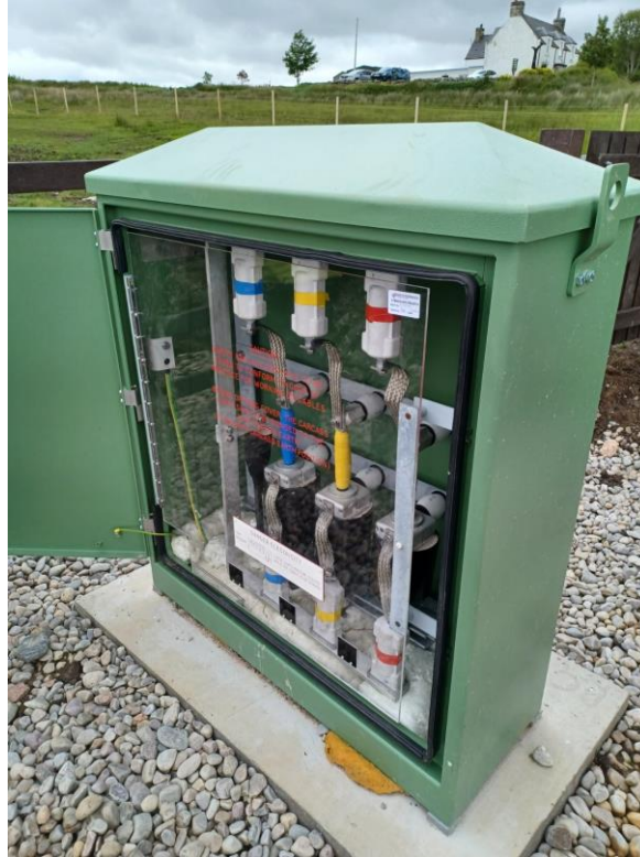
Plate 3.7: Typical Link Pillar
