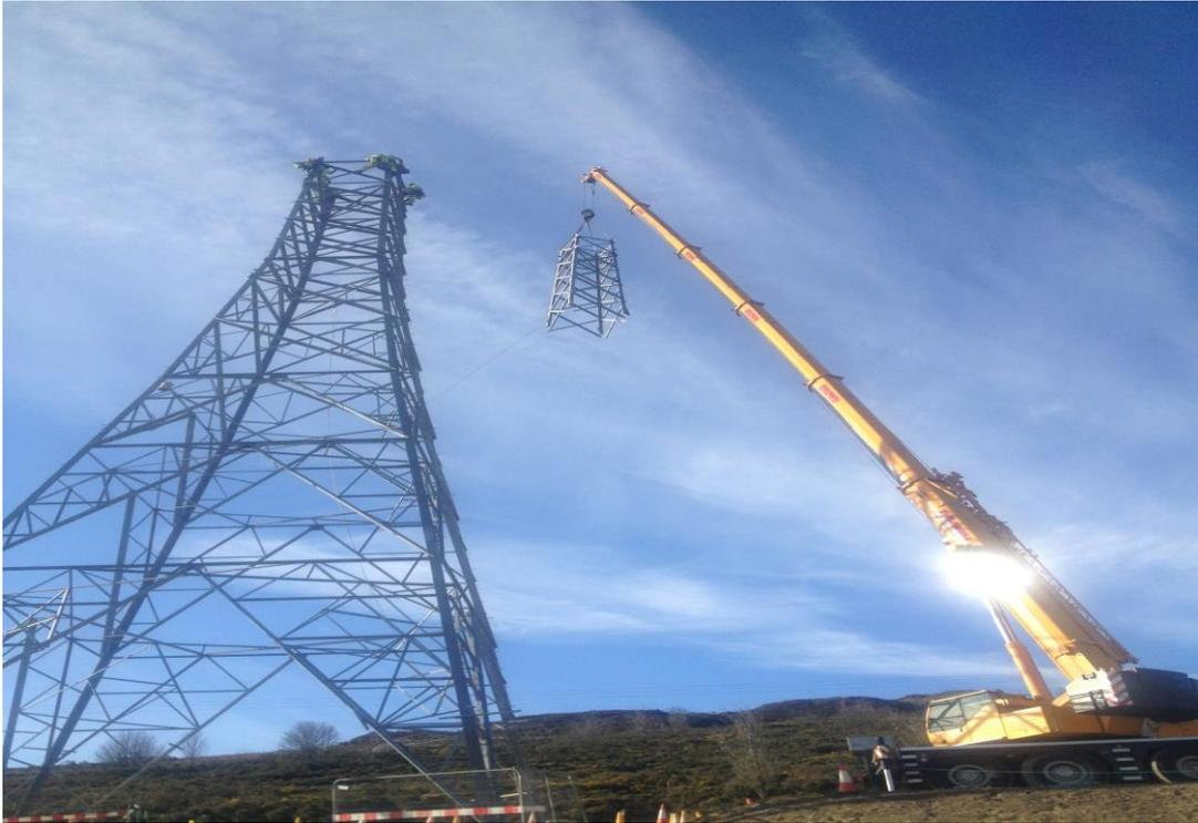
BBK – erecting a new tower on the 275kV line
