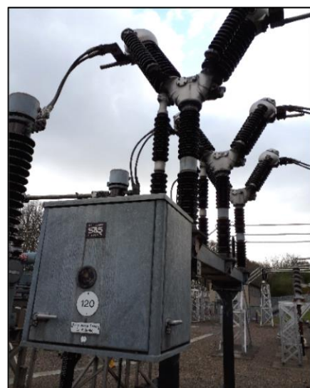
Figure 7 – 132kV AIS Circuit Breaker
