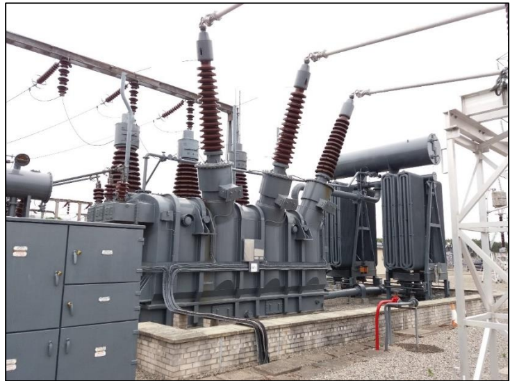
Figure 6 – 275, 120MVA Parsons Peebles SGT manufactured in 1970
