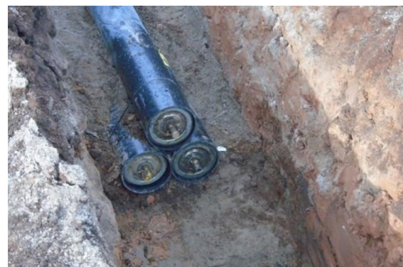
Figure 9 – 132kV XLPE Cable Installation
