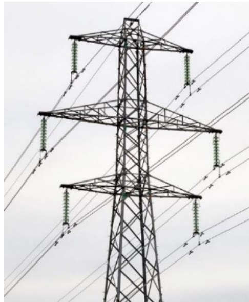
Figure 10 – 132kV Steel Lattice Tower & Wood Pole Lines
