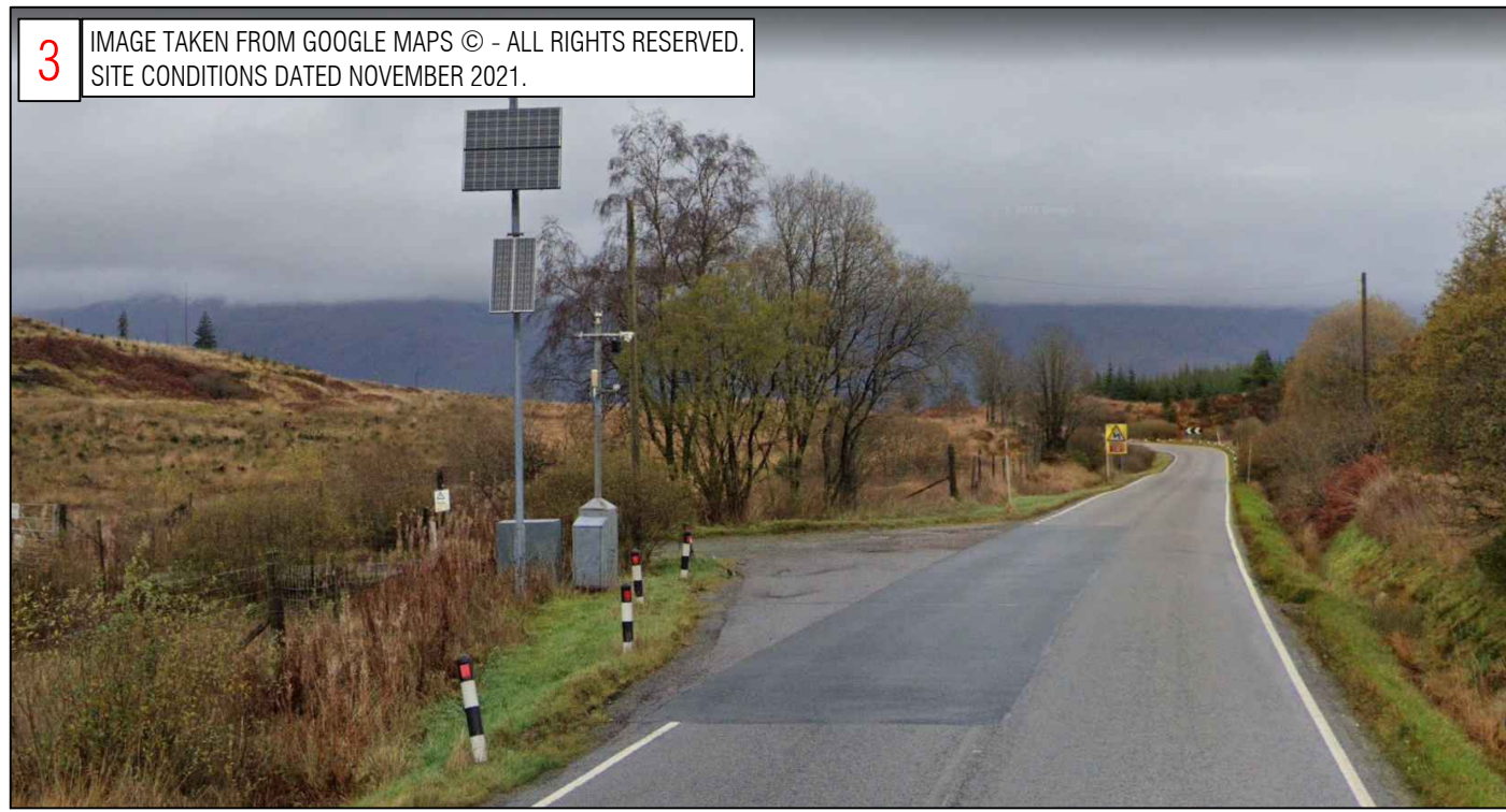
EXISTING SITE CONDITIONS (FROM NORTH)
