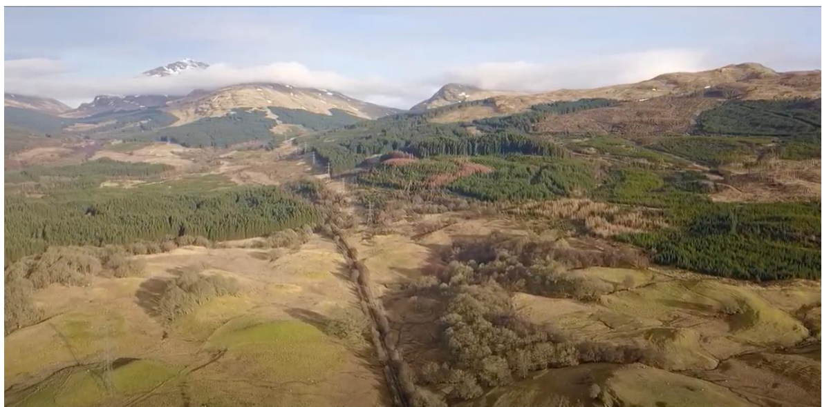
Plate 2.8: Drone view between T44-T47
