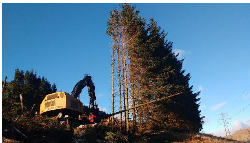
2 - Live overhead line techniques using Tigercat to remove trees that would otherwise require an outage due to the proximity of the transmission circuit to the right.
