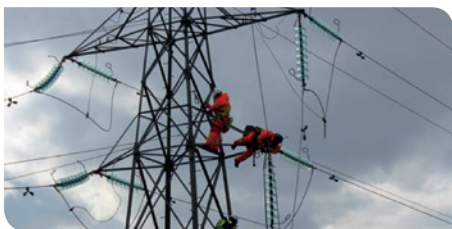
Work underway on the Fort Augustus to Fort William 132kV line
