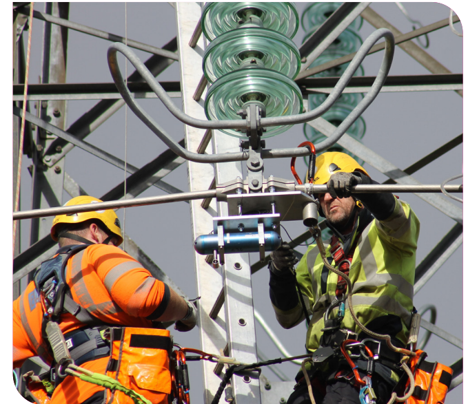
Engineers installing vibration monitoring equipment at Gordonbush
