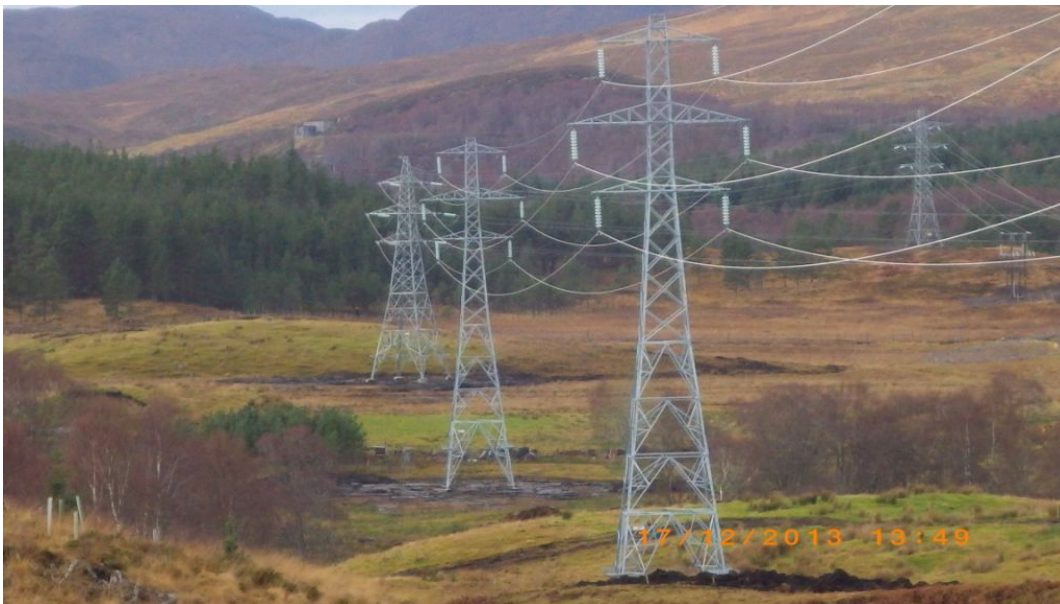
Beauly Mossford – new towers erected
