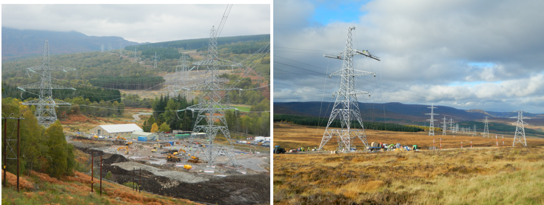
Beaully Denny – Tummel substation under construction and new conductors being installed
