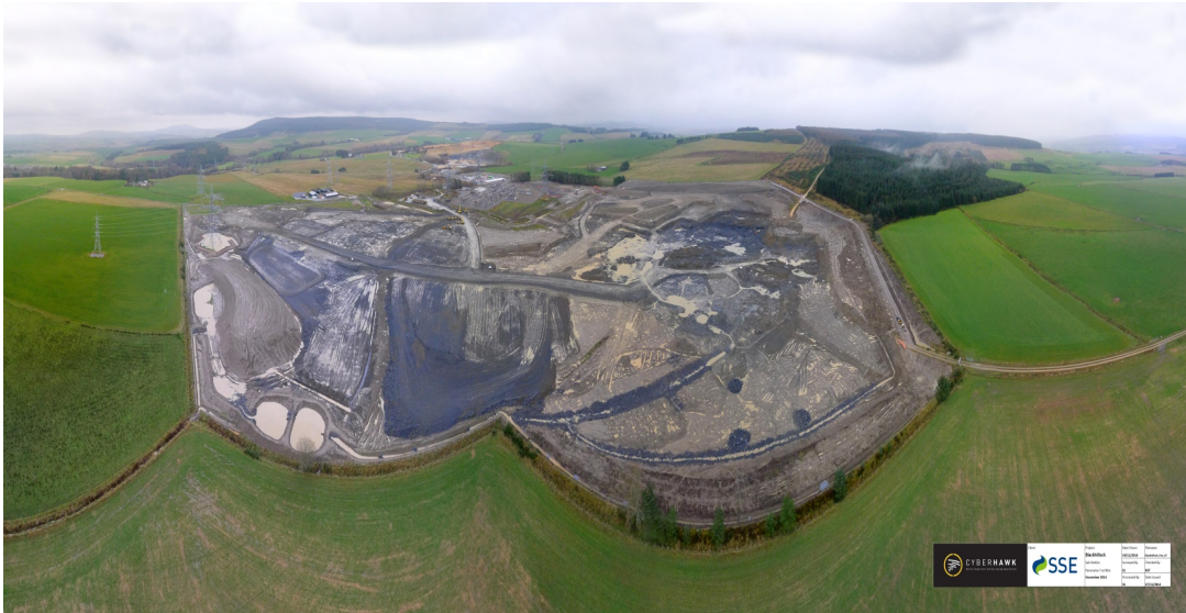
Caithness-Moray – Civil Construction Works at Blackhillock Substation
