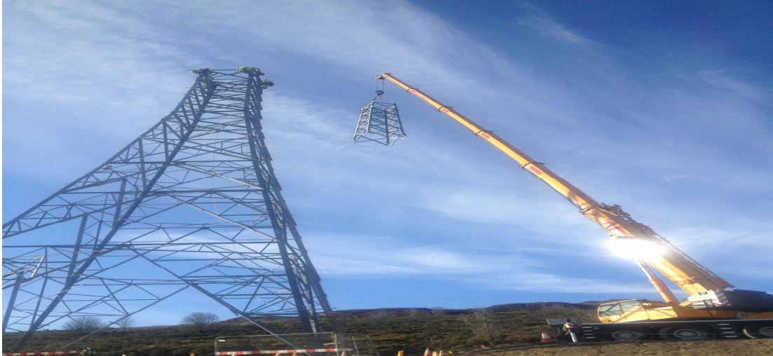
BBK – erecting a new tower on the 275kV line
