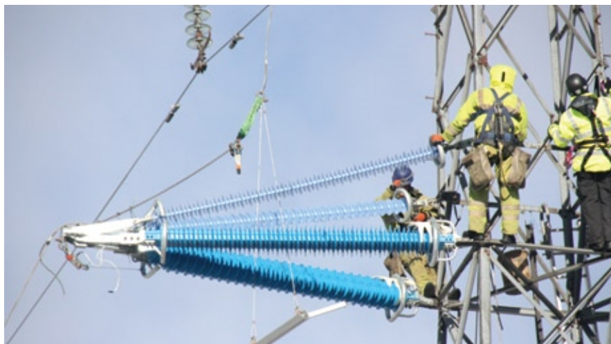
Figure A5.4 Installation of insulated Crossarms
