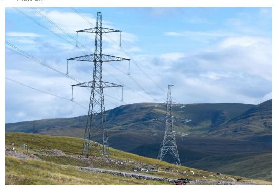
Plate 2.1 – Existing SSE400 steel lattice tower design
