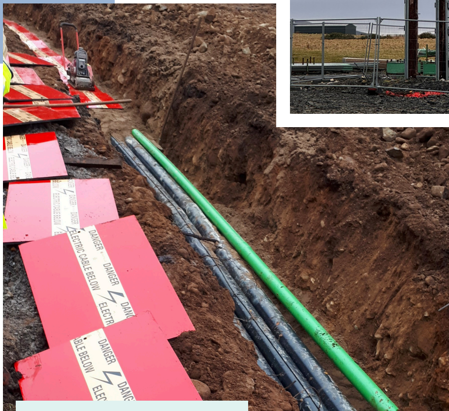
Typical 132kV cable trench arrangement
