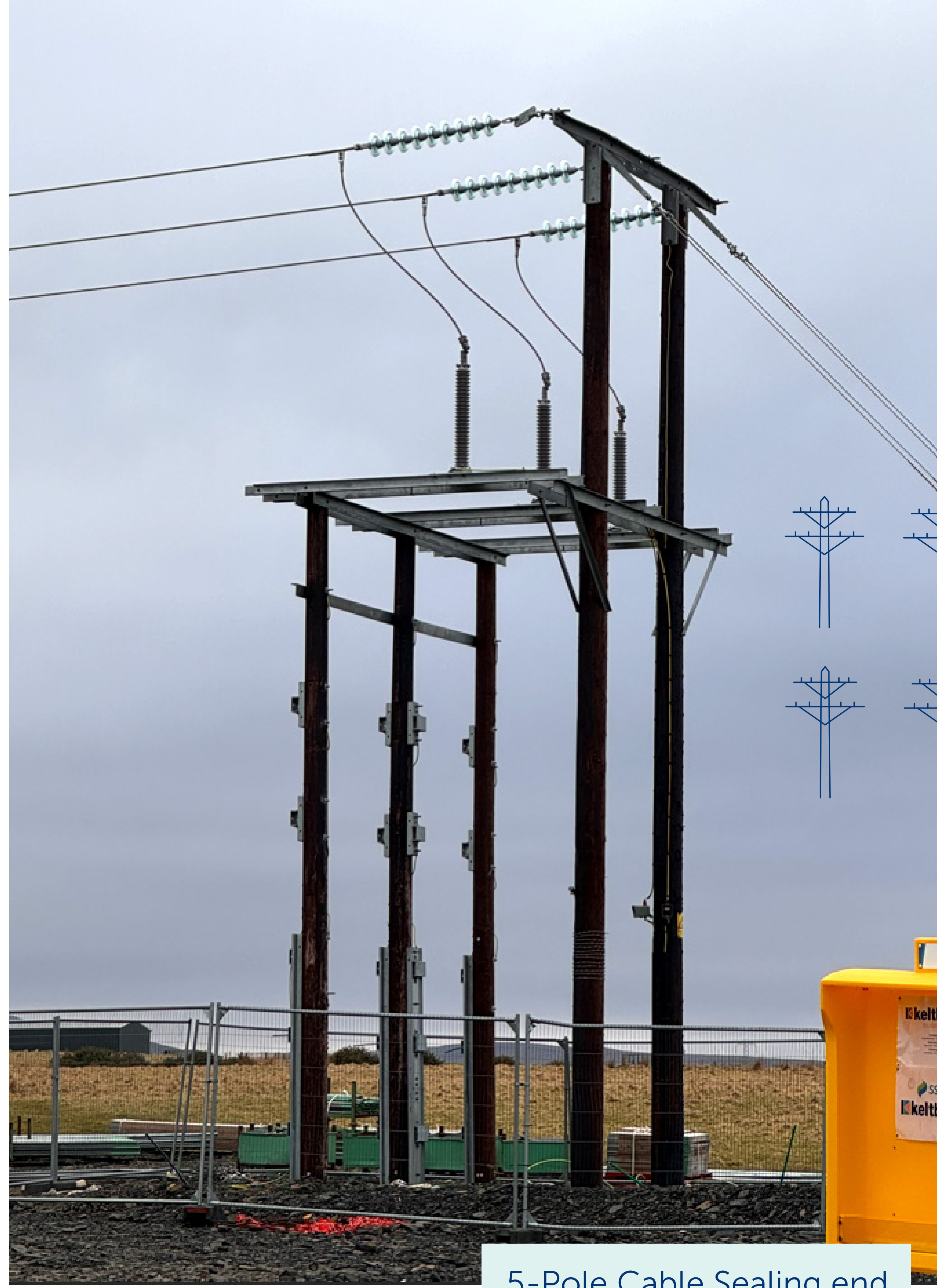
5-Pole Cable Sealing end
