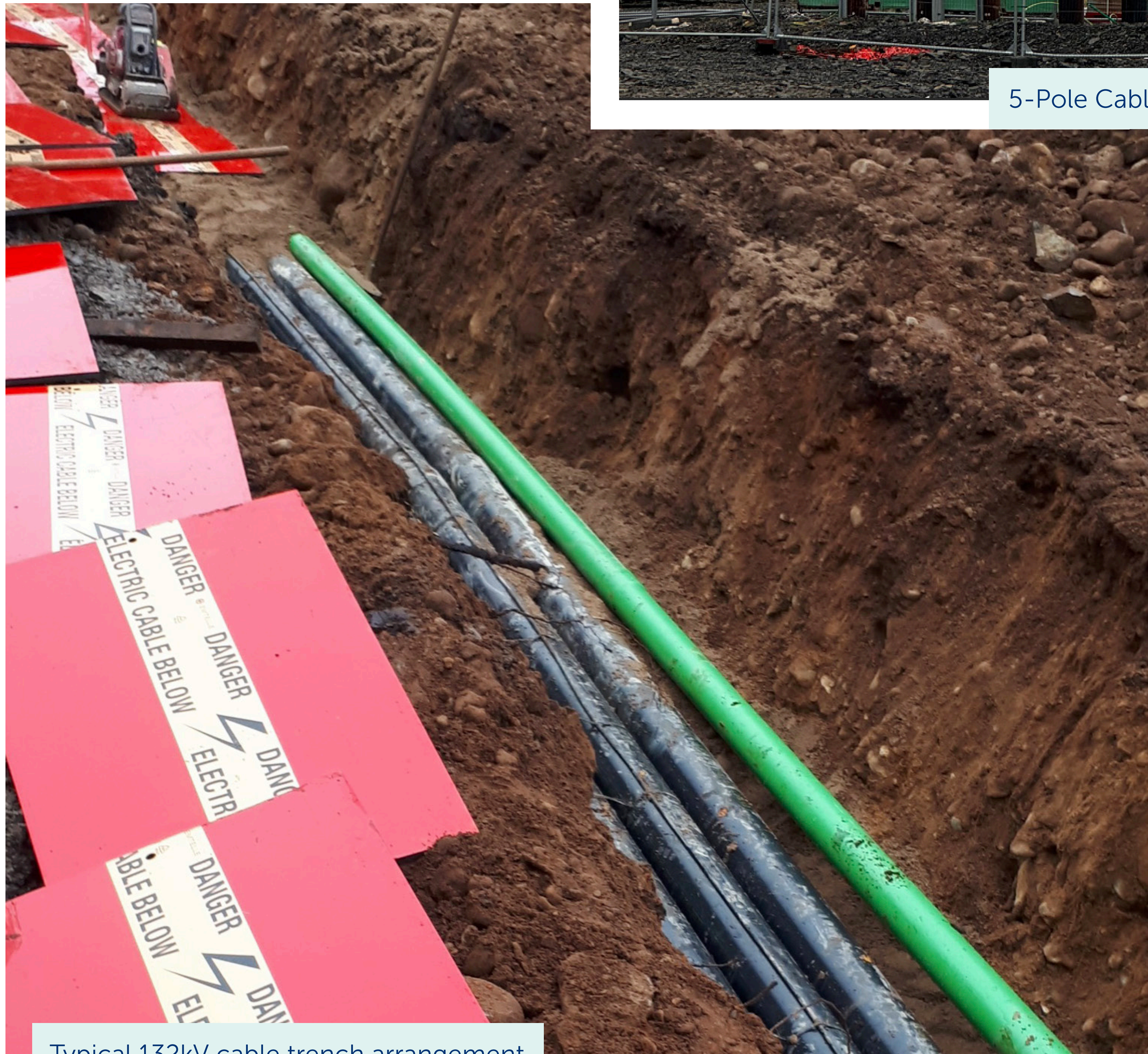
Typical 132kV cable trench arrangement
