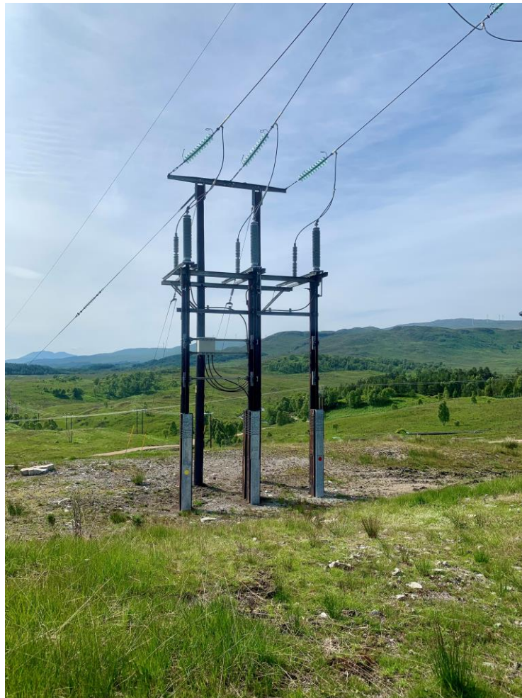
Plate 3.2: Typical Cable Sealing End Structure
