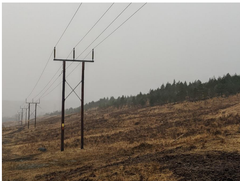
Plate 3.1: Typical H Wood Pole
