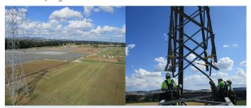
To date, our Principal Contractor, Balfour Beatty, who are delivering the OHL works, have completed the erection of the two temporary towers required to create a temporary bypass. Both towers are located adjacent to the existing overhead line.
