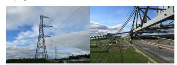
The temporary bypass that is required to enable the new permanent towers to be constructed has been completed. The above pictures show one of the temporary towers and linesmen connecting insulators from the temporary tower to the cross arm of one of the existing towers.
