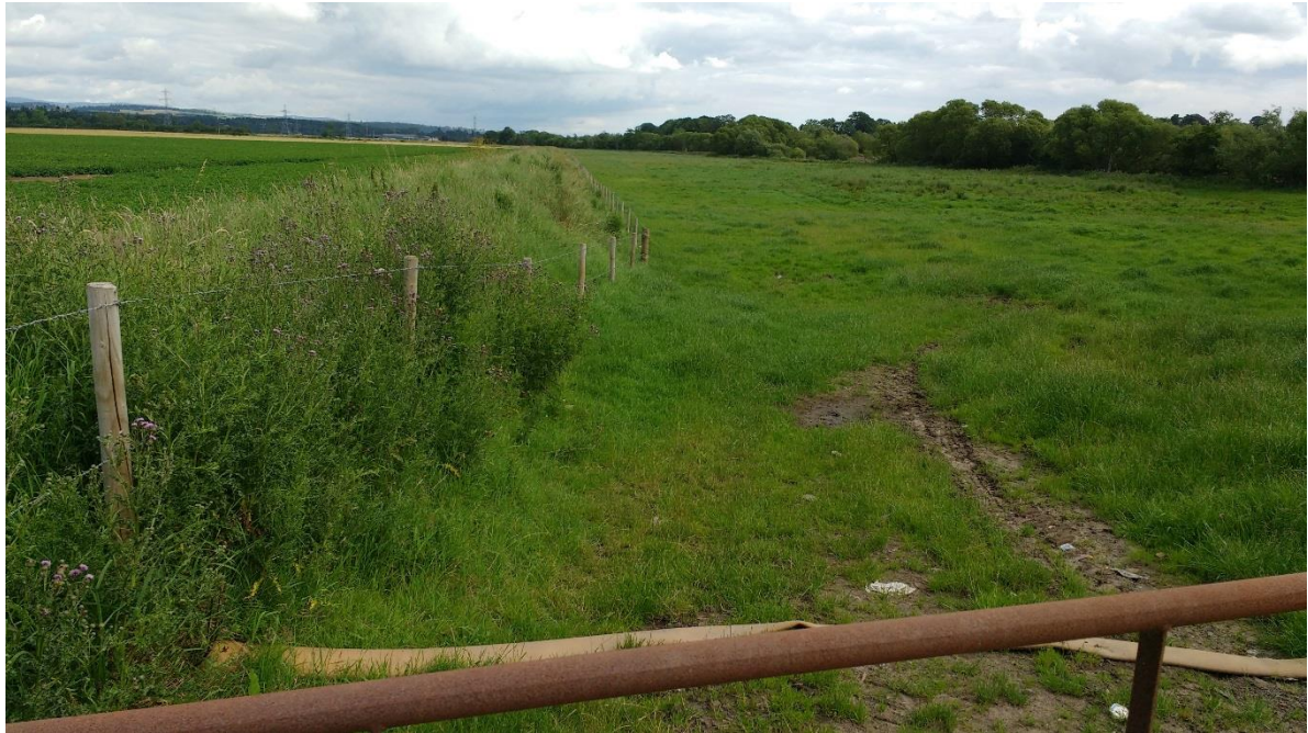
Photograph 7-6 – Linear Embankment Along River Isla Floodplain
