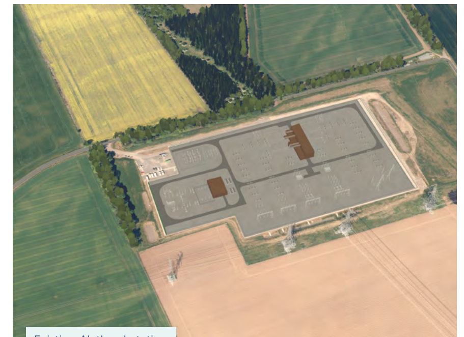
Existing Alyth substation
