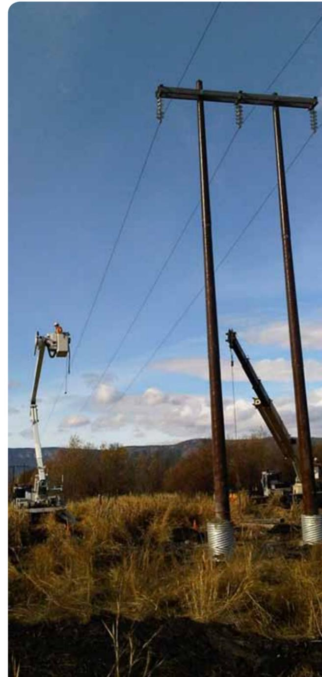
Due to the length of crossing at Loch na Deasport and Loch Ulapuil, where a wooden H pole does not have the capacity to support the span of conductor required, it is proposed to use composite poles at these two locations. Composite poles can be constructed of resin infused fibre glass or using steel poles with composite fittings.
