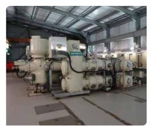
An example of standard 132kV GIS equipment housed inside a Switching Station.
