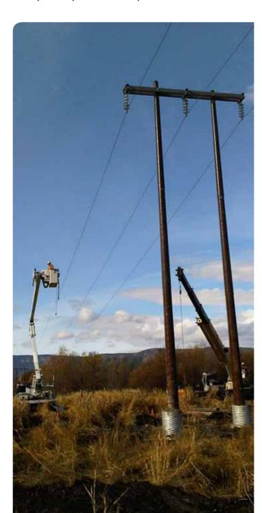
Due to the length of crossing at Loch na Deasport and Loch Ulapuil, where a wooden H pole does not have the capacity to support the span of conductor required, it is proposed to use composite poles at these two locations. Composite poles can be constructed of resin infused fibre glass or using steel poles with composite fittings.
