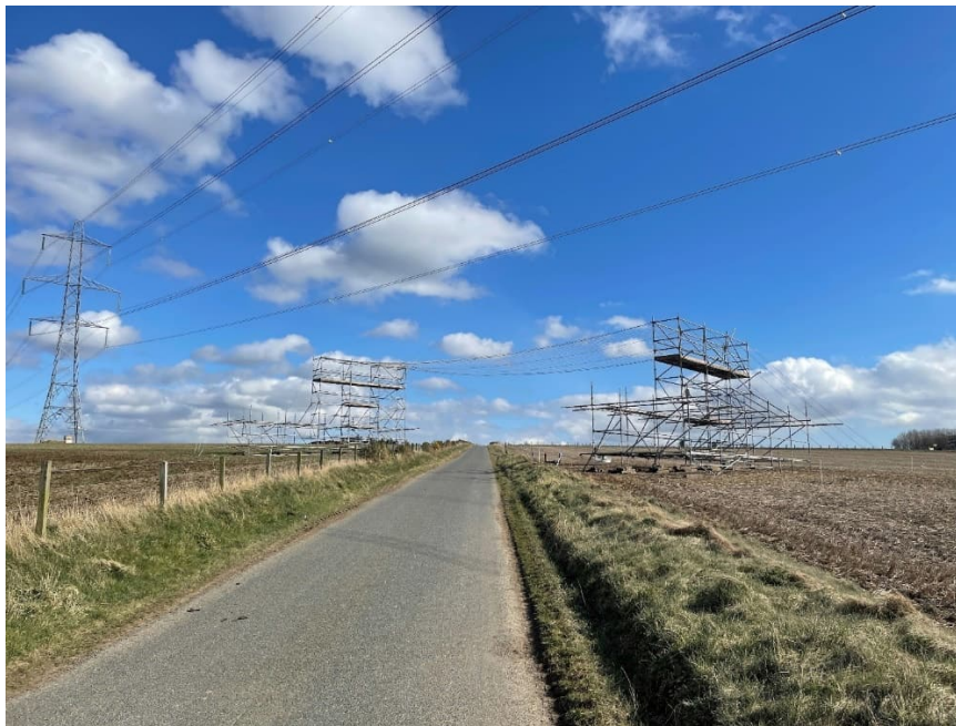
Plate 7: Illustrative Image of Temporary Construction Scaffolds
