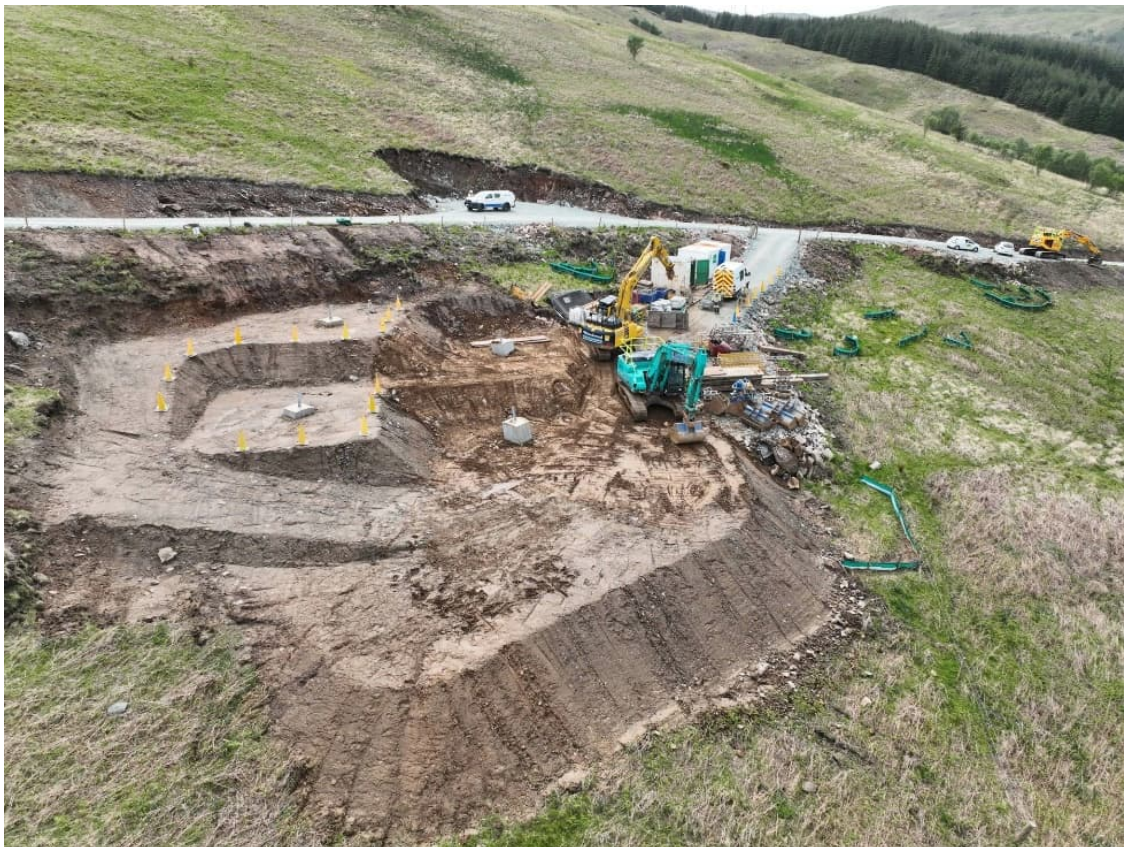
Plate 5: Illustrative Image of Tower Foundation Construction
