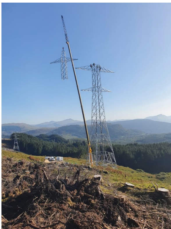
Plate 6: Illustrative Image of Tower Construction
