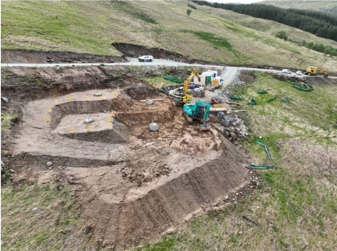
Plate 3.2: Illustrative Image of Tower Foundation Construction
