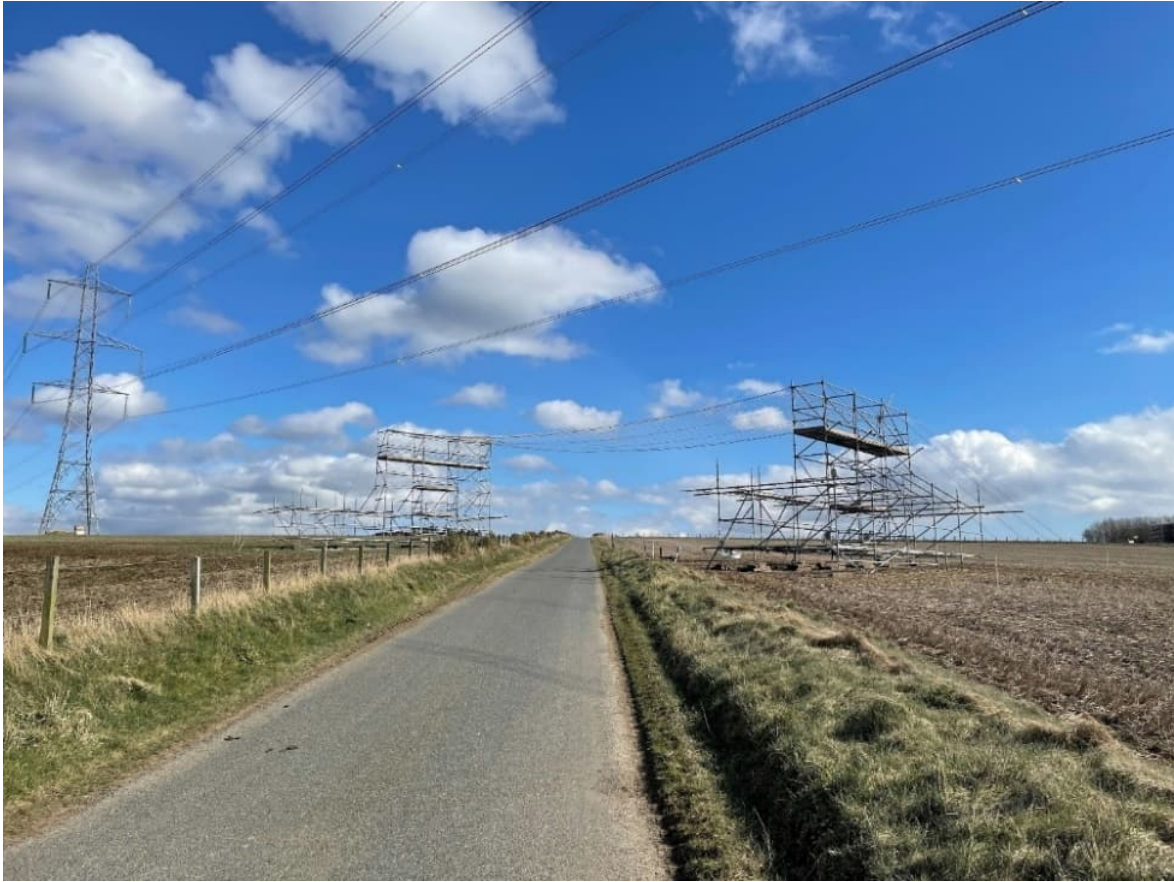
Plate 3.3: Illustrative Image of Temporary Construction Scaffolds
