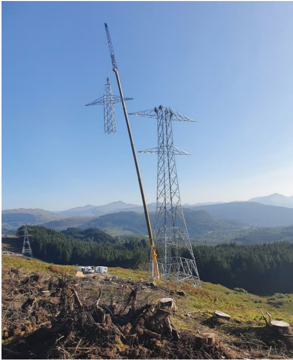
Plate 3.5: Illustrative Image of Tower Construction
