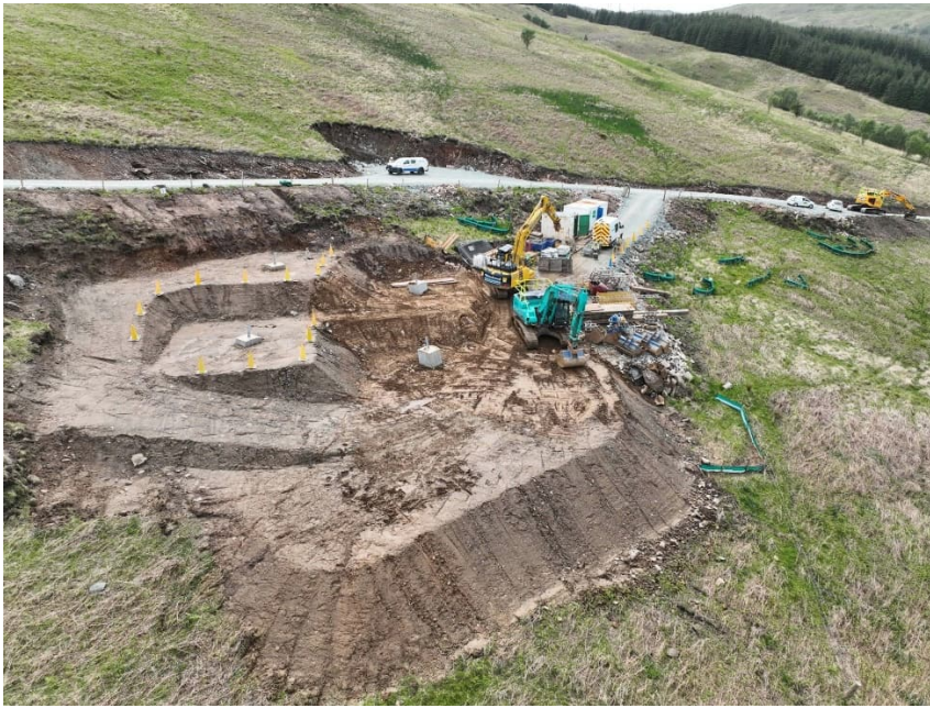
Plate 3.4: Illustrative Image of Tower Foundation Construction
