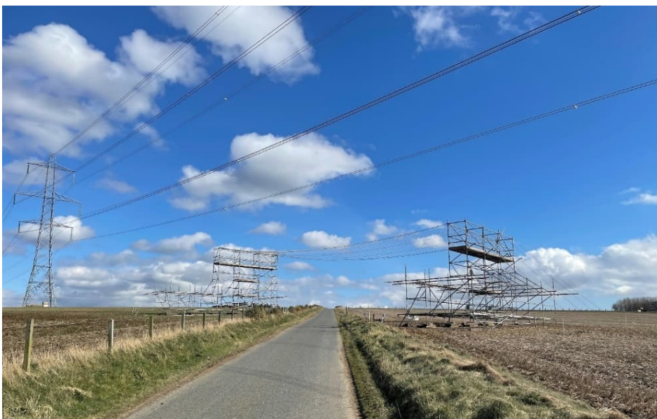
Plate 3.6: Illustrative Image of Temporary Construction Scaffolds
