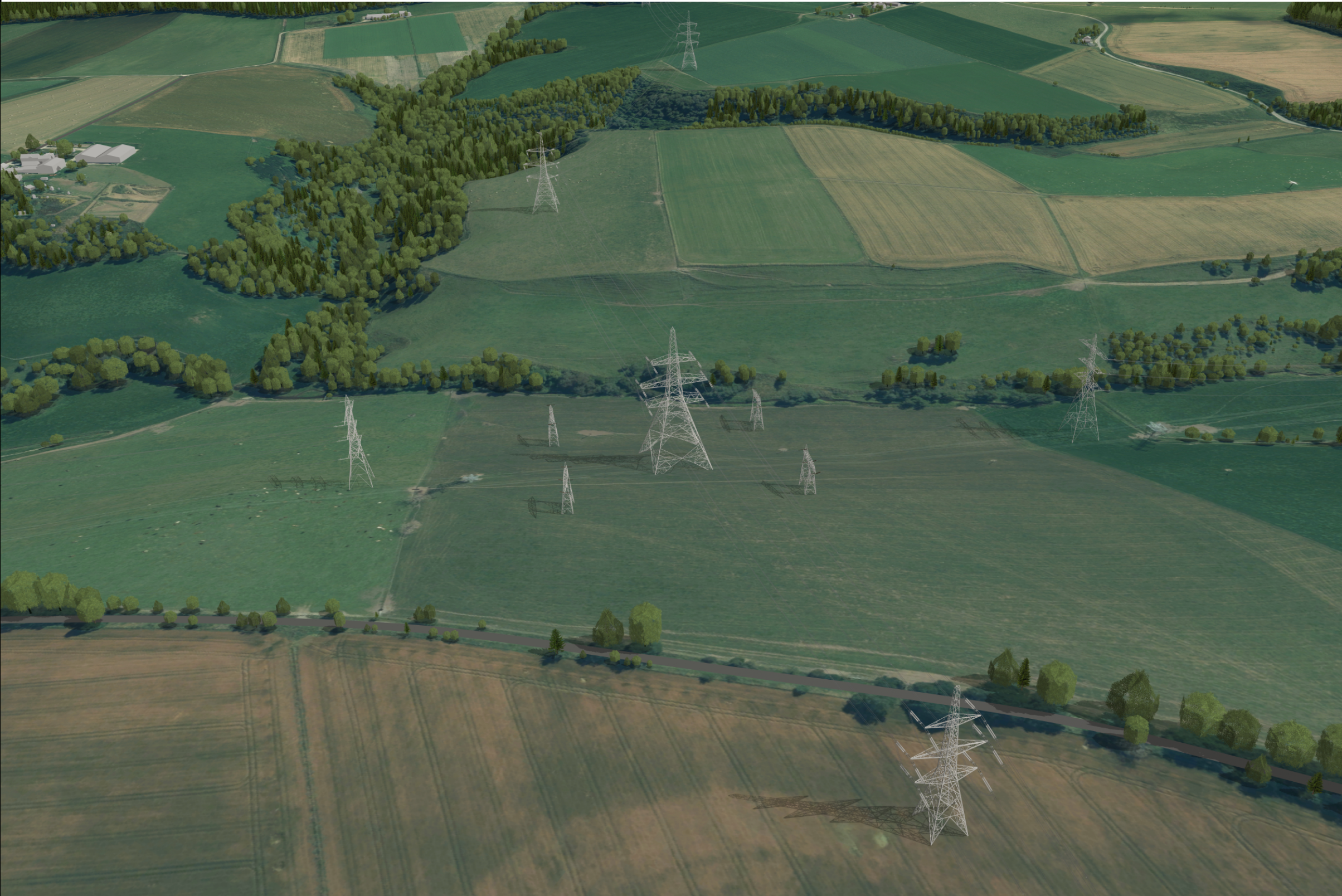
Existing OHL Crossing 5
