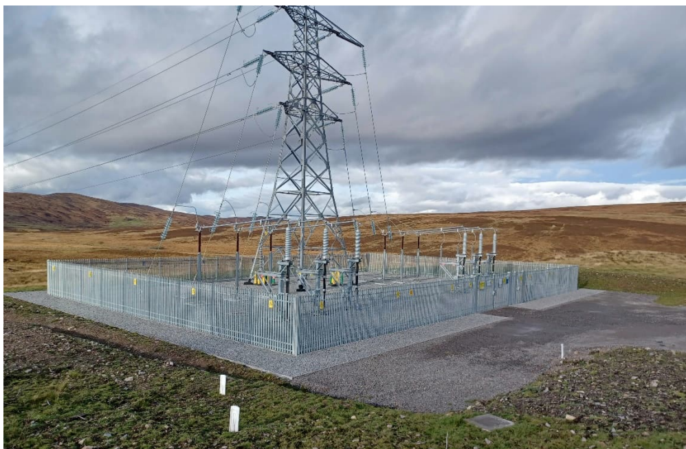
Plate 2.2: Example of a Cable Sealing End Compound
