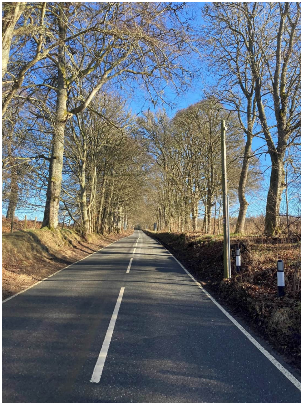
Photo 4: View at NH 633751 401213 looking northeast on the B862. Showing mature broadleaved avenue of trees.
