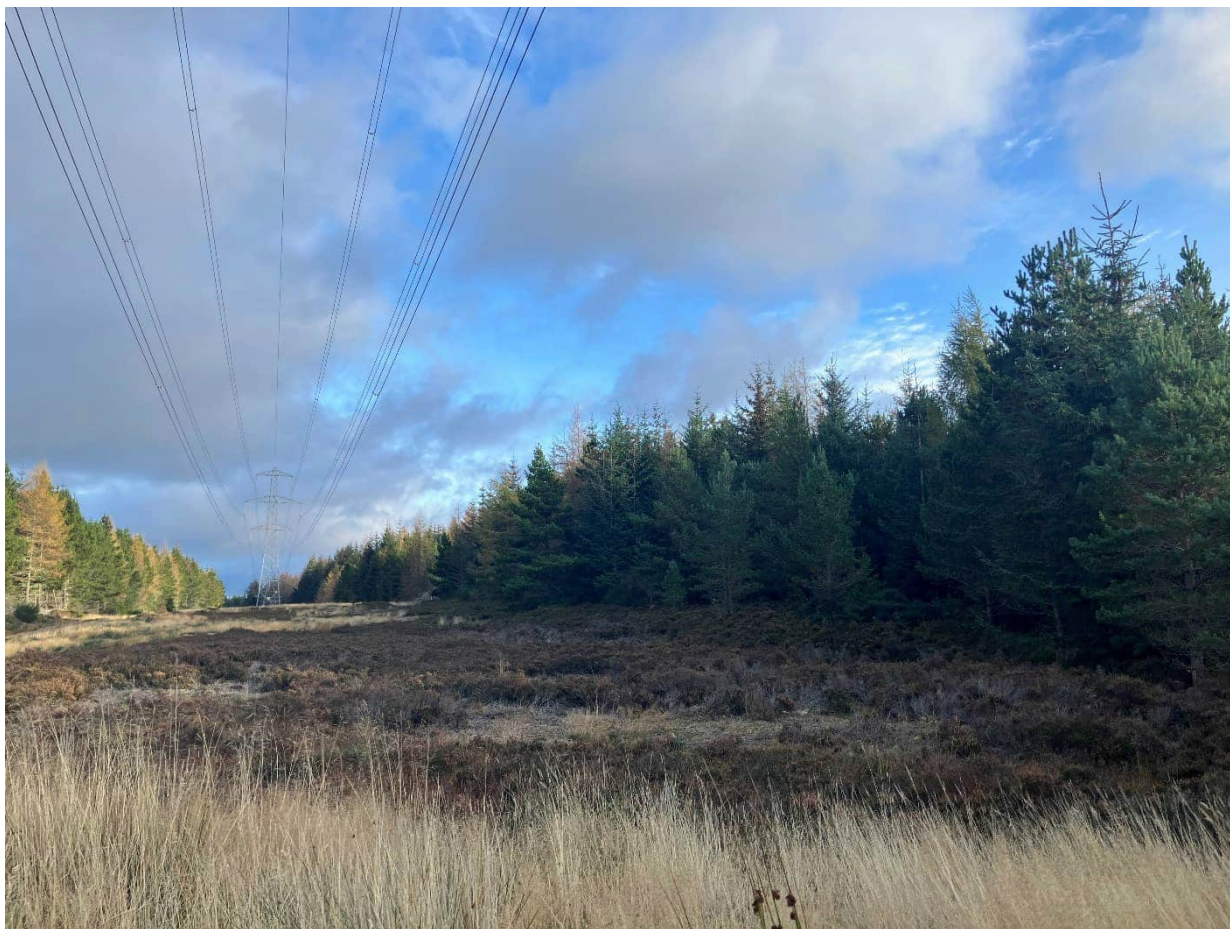
Photo 1: Existing OHL with green edges, proposed new line to run parallel on right hand side (NH 696533 399817, looking northeast)
