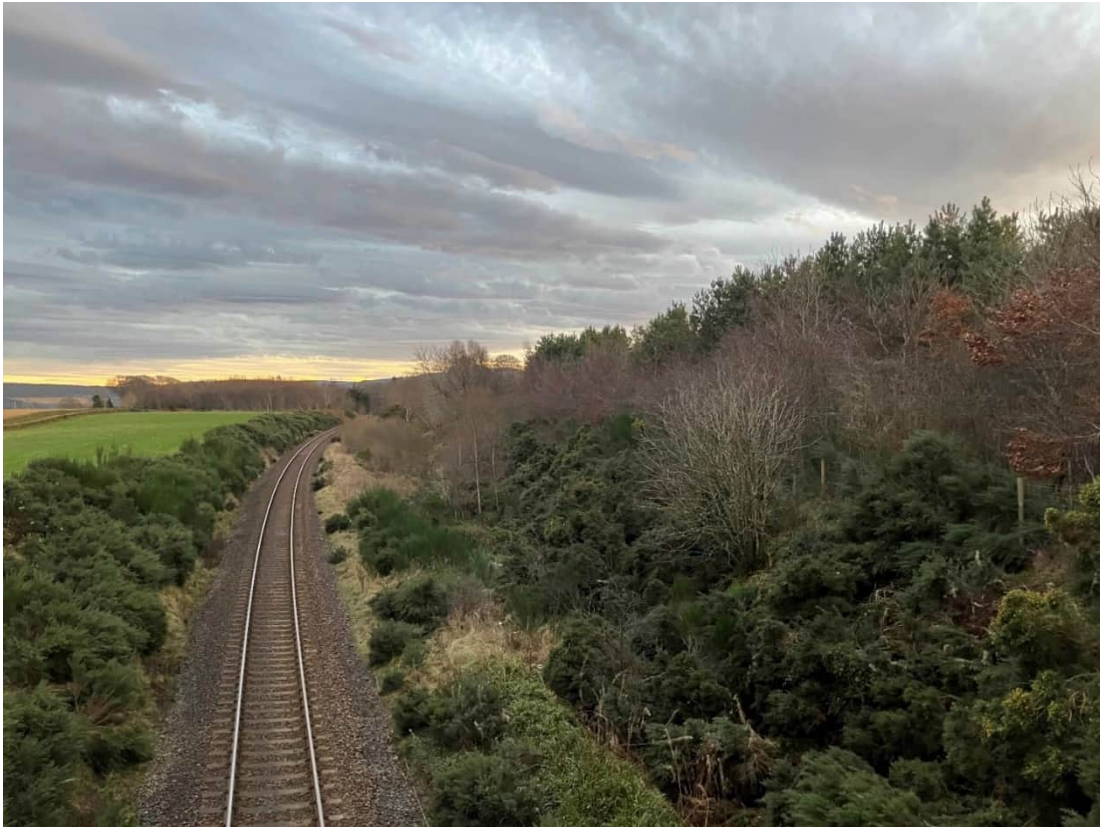
Photo 1: Sporadic natural regeneration along railway line looking south (NJ 305345 580421, looking southwest)
