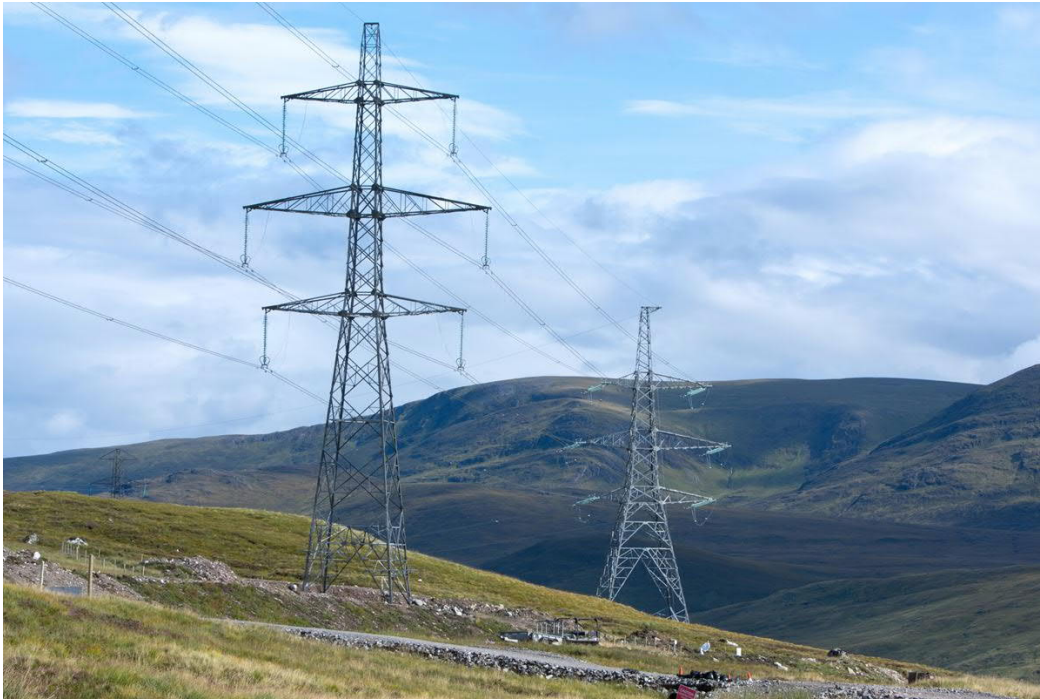
Plate 2.1 – Typical SSE400 steel lattice tower design
