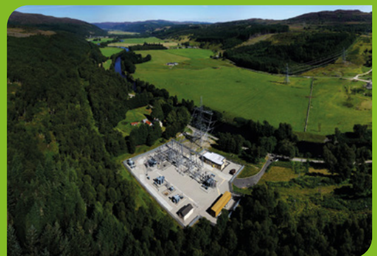
Existing Fasnakyle 275kV Substation
