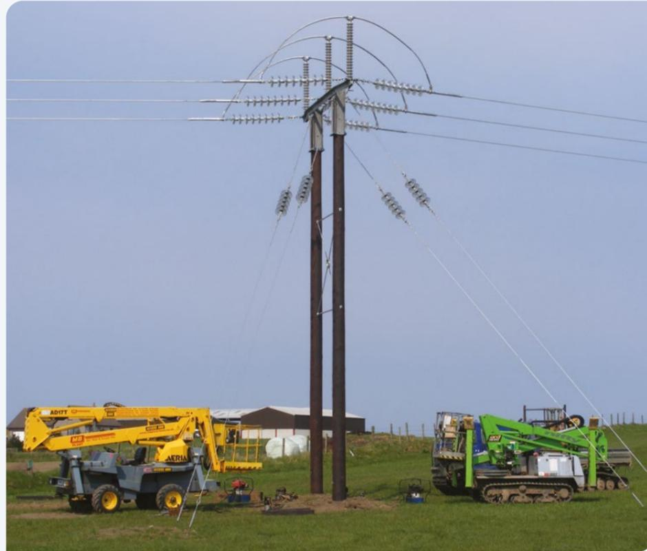
Above is a typical example of an angle wood pole which requires additional stays. Note that stays are not usually required on non-angle poles unless ground or weather conditions dictate.
