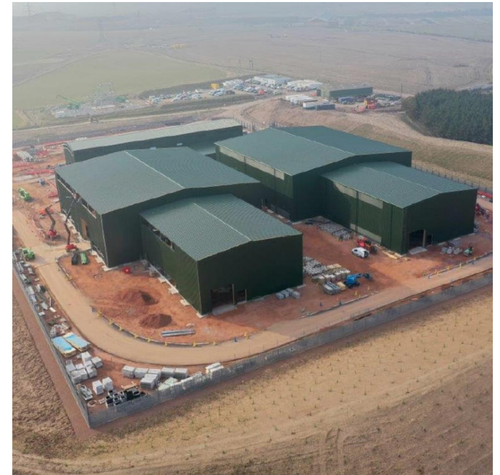
The 400kV GIS substation at Peterhead
