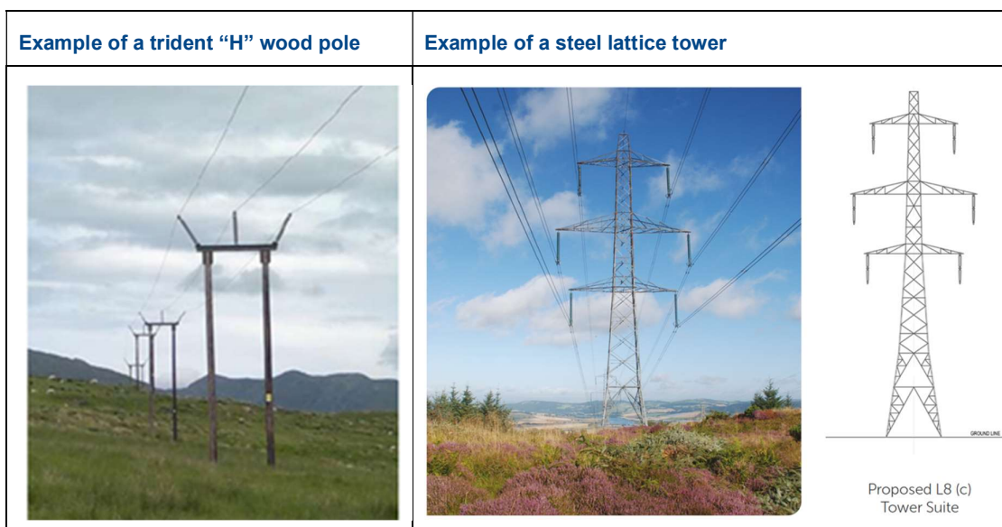
Plate 1: ‘H’ Trident Wood Pole and Steel Lattice Tower examples.
