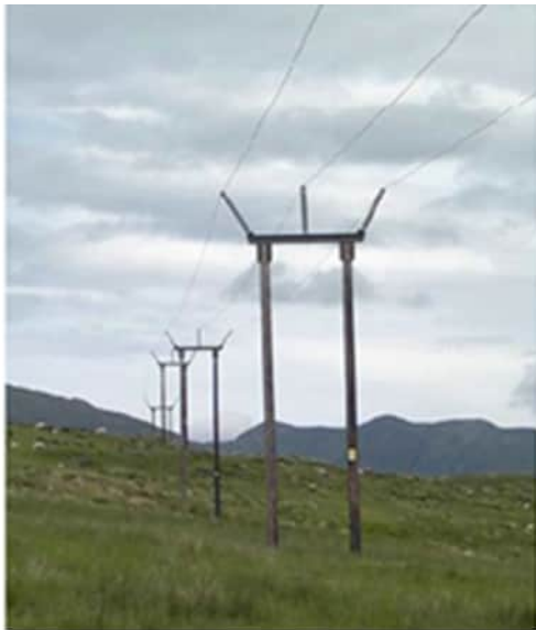
Photograph 2.1: Indicative Trident 'H' Pole Example
