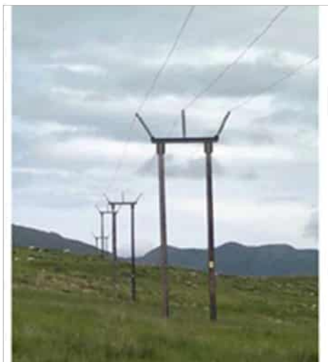
Photograph 2.1: Indicative Trident 'H' Pole Example
