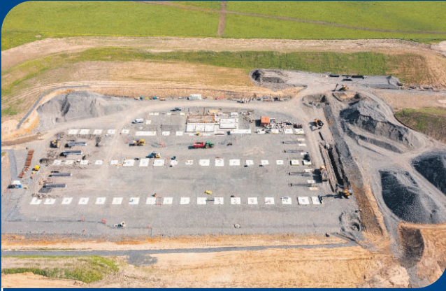
June 2021 - platform complete and foundations nearing completion.
