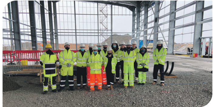
The Rolls Royce Vulcan apprentices at the Switching Station development and were provided an update on the project progress.
