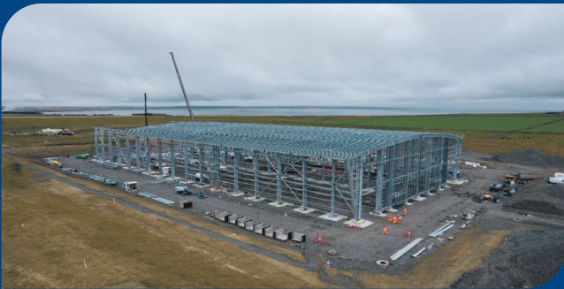
August 2021 Main steel work complete.
