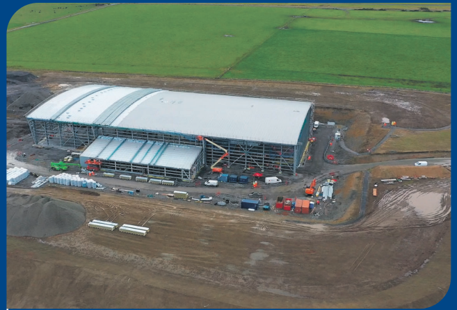
Roof cladding underway, October 2021.
