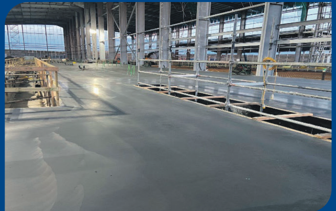
November 2021 reinforcement concrete floor slabs 80% complete.
