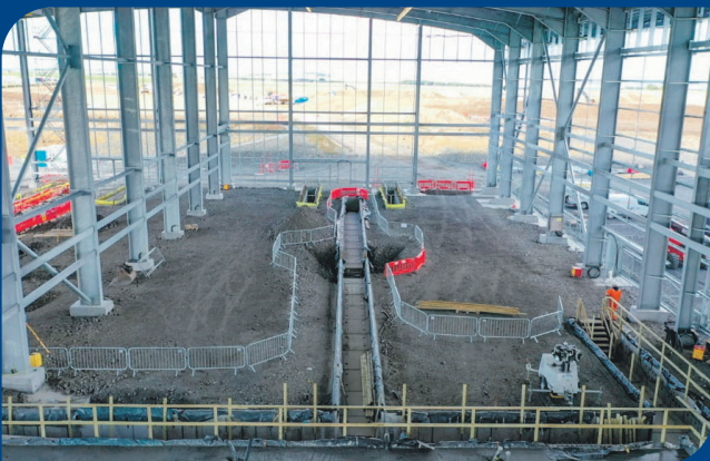
September 2021 Precast cable trough installed.
