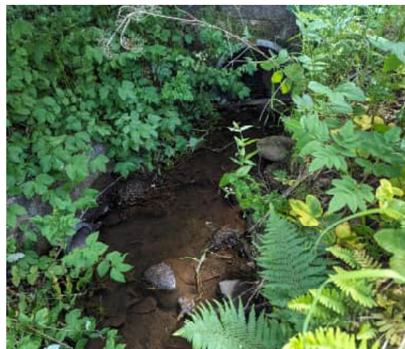
Plate 9-7 Taken at NN 83185 09095 facing downstream at culvert at the B8033 on 11 June 2024
