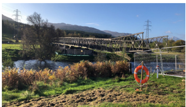
Example of a Bailey bridge used on a nearby SSEN Transmission project at Killin which would be used for the haul road crossing the Keir Burn.
