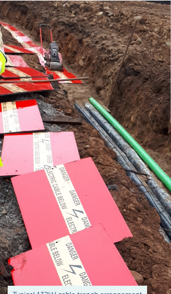
Typical 132kV cable trench arrangement
