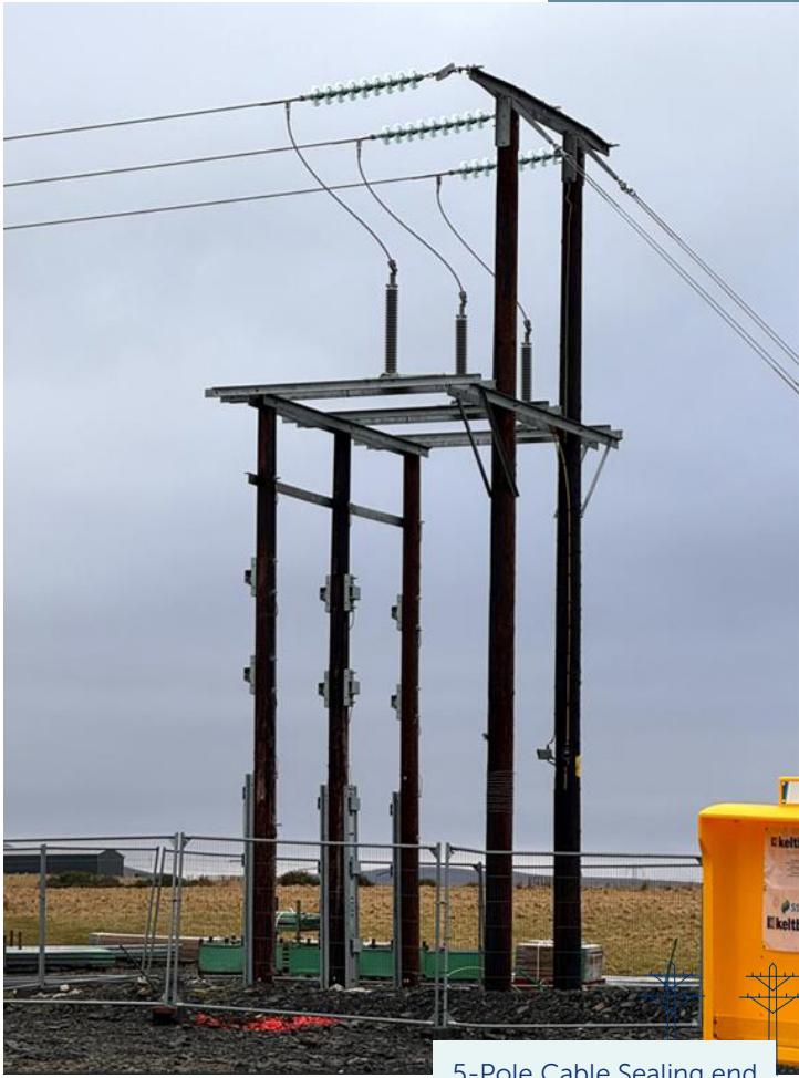
5-Pole Cable Sealing end
