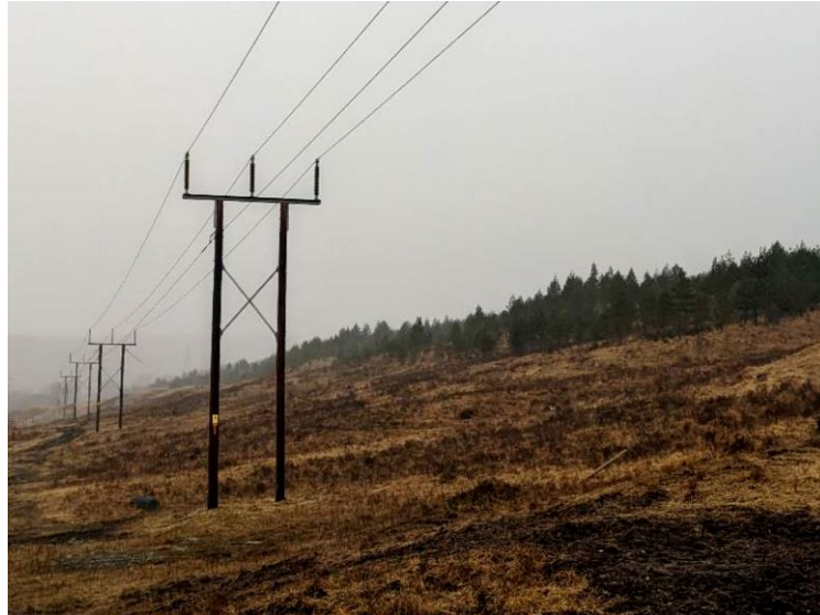
Plate 2.1 – Typical wooden trident pole design
