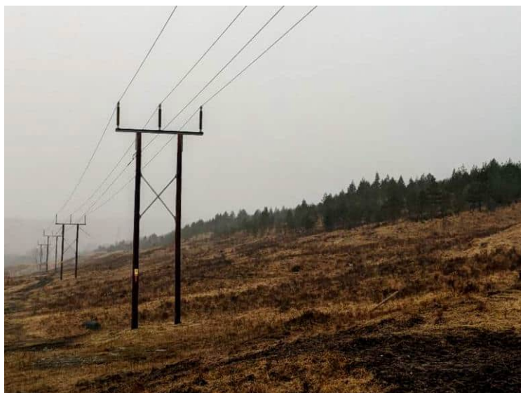
Plate 2.1 – Typical wooden trident pole design
